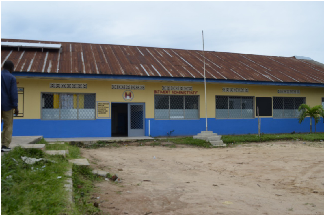
Administrative and laboratory building
